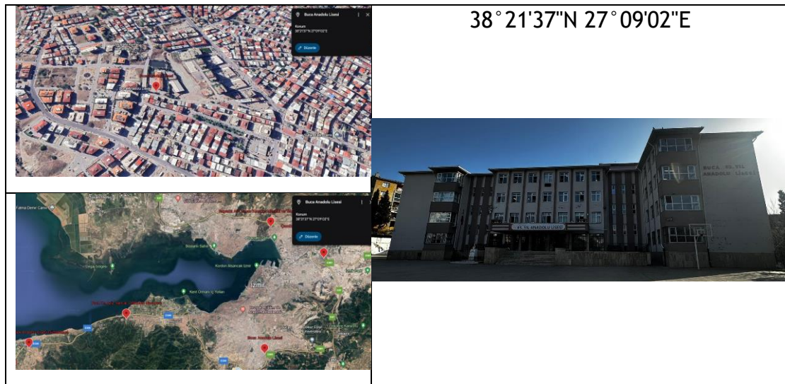
Figure 105. Google map view, geographical coordinates and a general photo of Buca Anadolu Lisesi.
