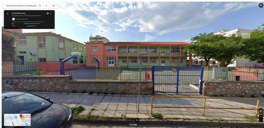
Figure 36. School building in Alexandroupolis, visually inspected using street view of Google maps.
