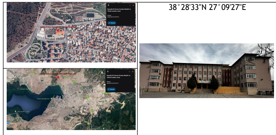
Figure 102. Google map view, geographical coordinates and a general photo of Ali Osman Konakçı Mesleki ve Teknik Anadolu Lisesi.
